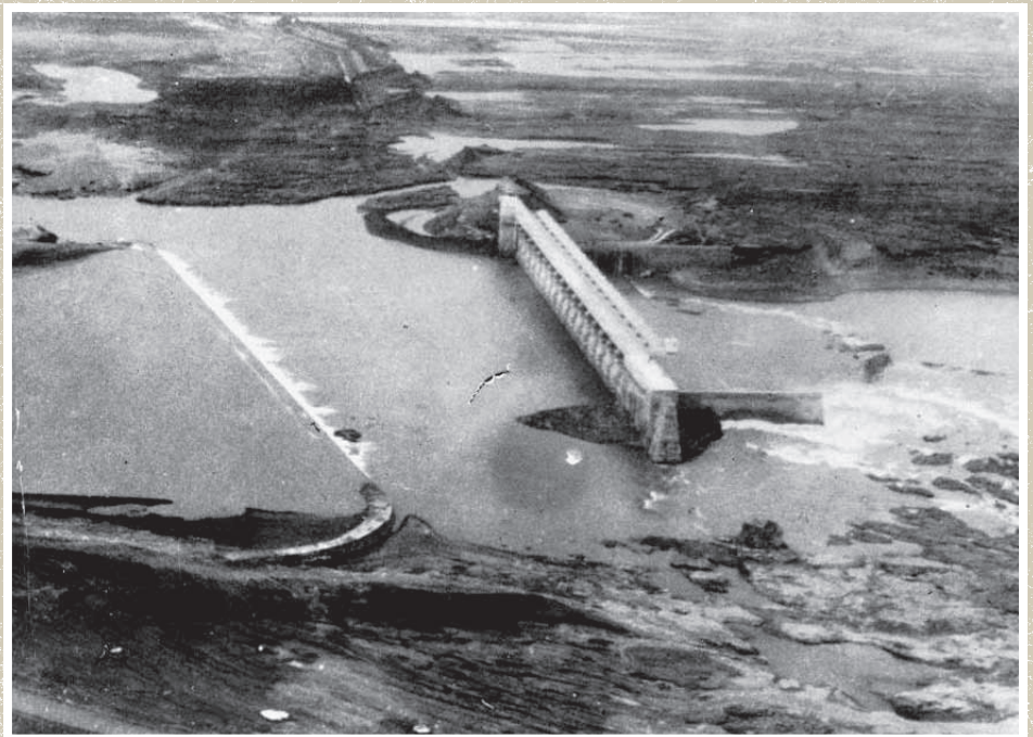
An aerial photograph of the Machhu Dam-II after the disaster.
